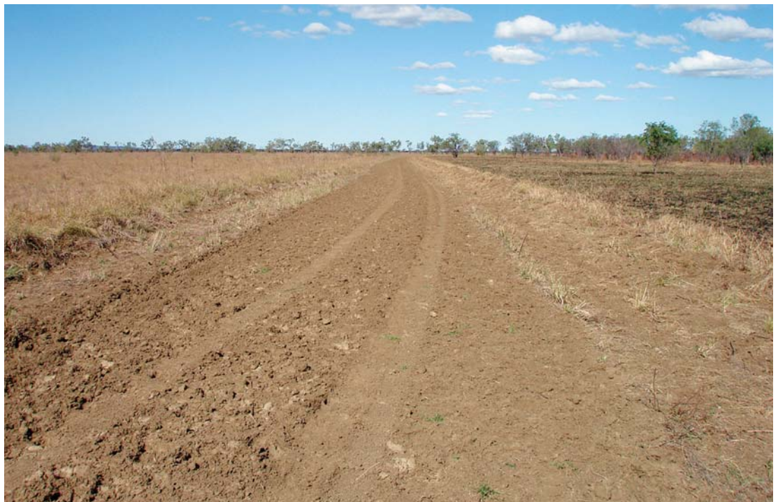
Figure 1. Mineral earth graded firebreak.
