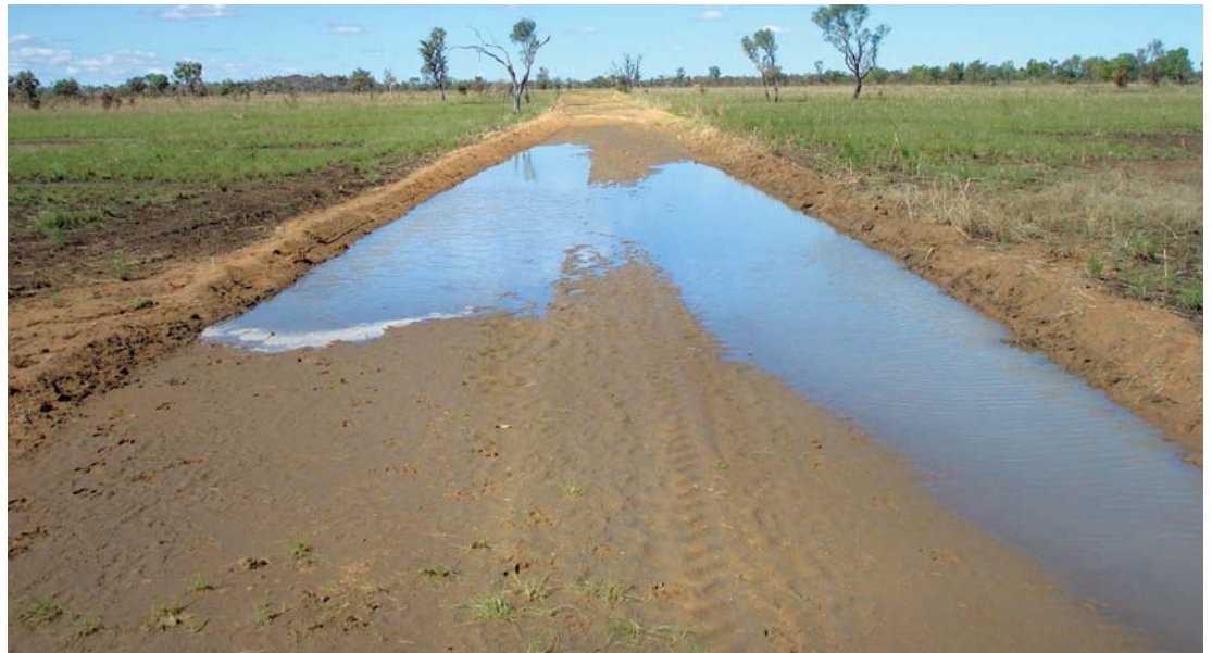
Figure 6. Water trapped on the firebreak because of the construction and the lie of the land.
